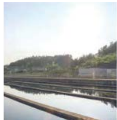
Urban Water Supply
